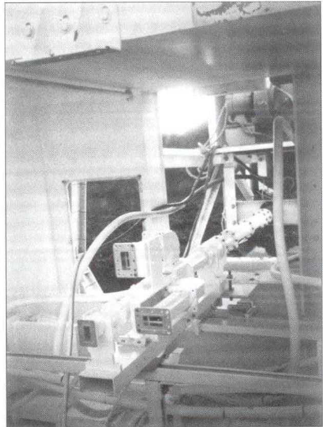
Figure 14. New 4/6-GHz feed for Santa Paula earth station provides low off-axis cross polarization
